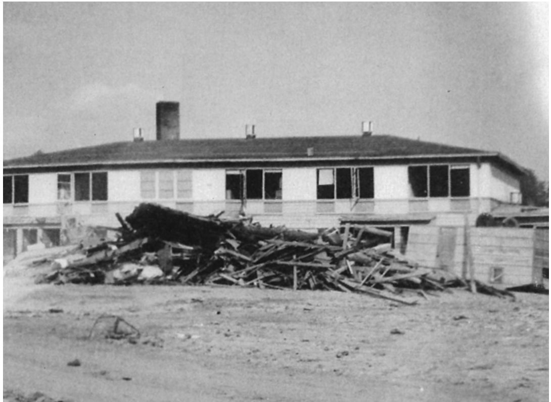
Our apartment building after the flood. Photo courtesy of V. Ballard.
