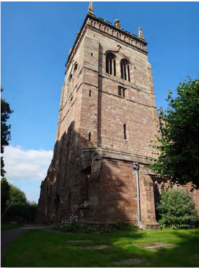
The bell tower at St. Mary's Church, Acton, Cheshire, England. The parish register states a storm blew down the tower on 15 March 1757. Brick repairs are shown above the old stone. Photo courtesy of the author.
