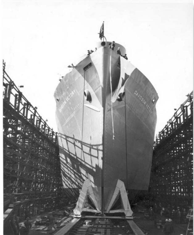
SS Davidson Victory on ways at Oregon Shipbuilding Corporation in March 1945. Davidson College/Oregon Shipbuilding Corporation. Wikipedia .
