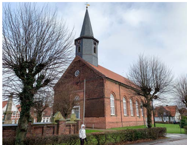
St. Wulphardi Church, Freiburg, Germany.
